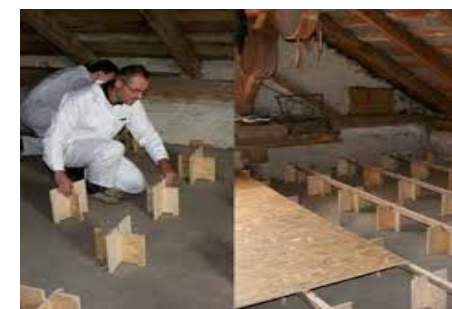
pose double plancher
