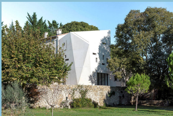
Extension maset Archi. : Dixneufcentquatrevingtsix Photo : F. Kleinfenn
