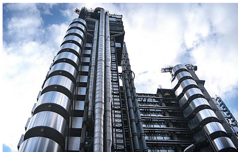
Lloyd's building Bank, Londres, Richard Rogers, 1984
