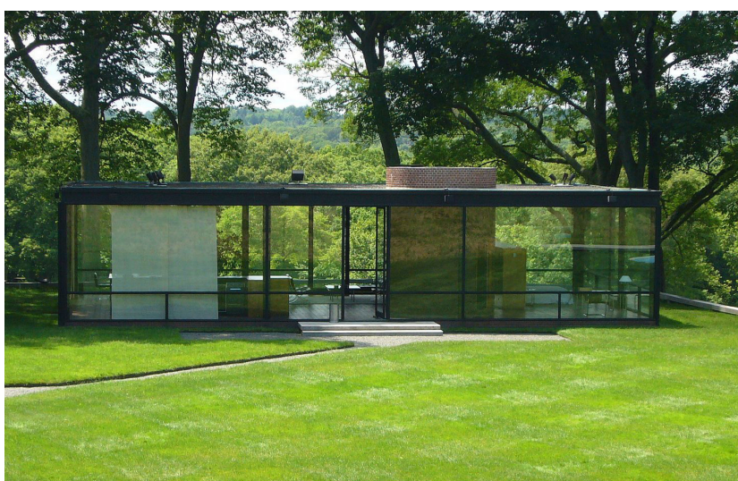
Glass House, New Canaan, Connecticut, Philip Johnson, 1949
